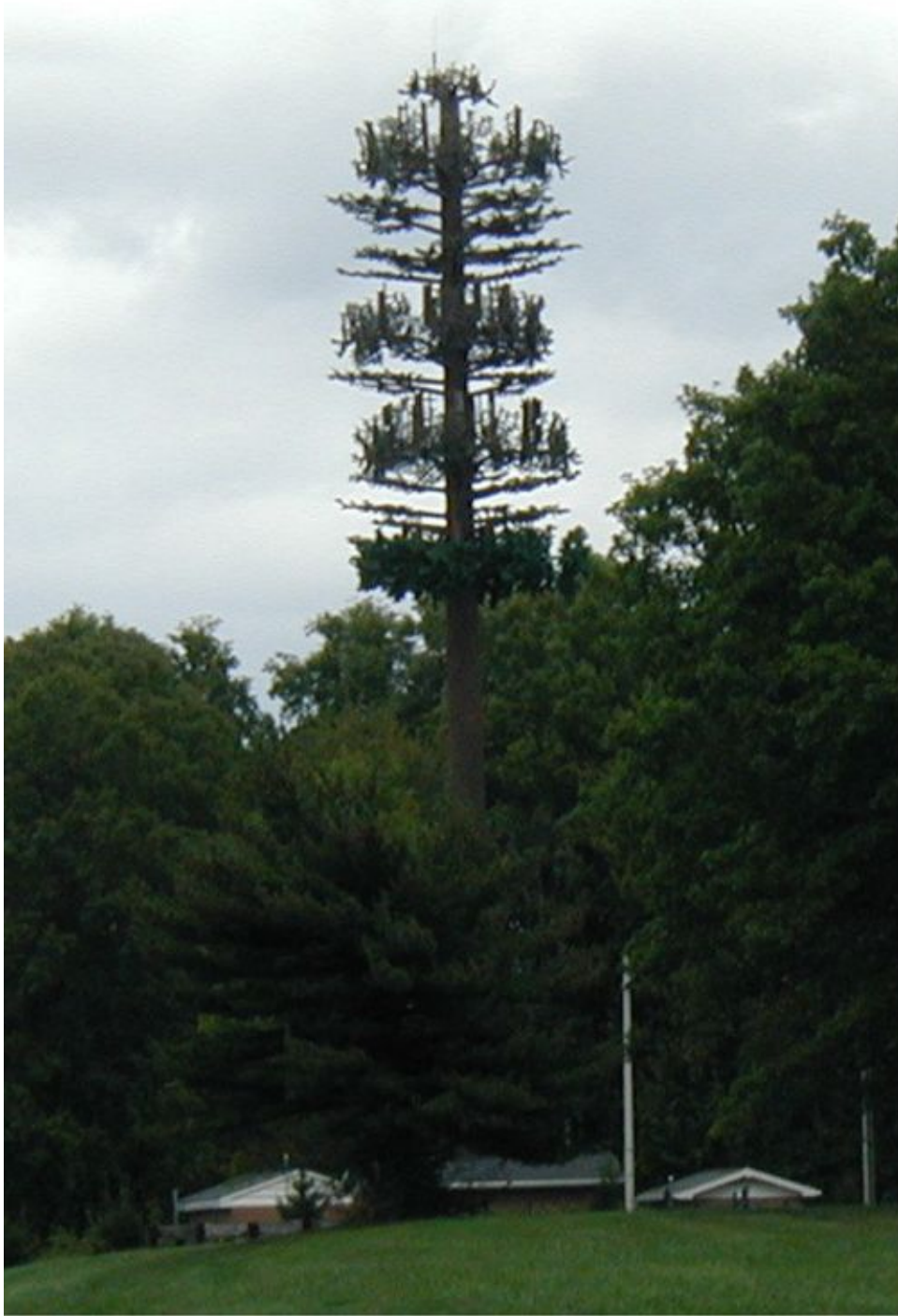
Figure 8.3: Cell phone tower disguised as a tree.
